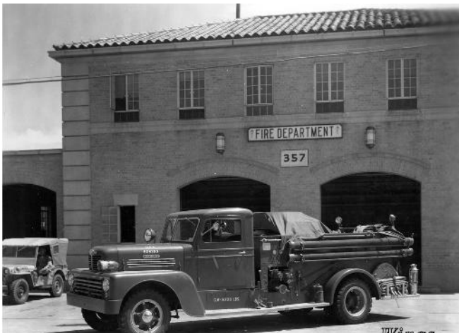
Fire Department – Building 357
