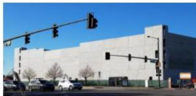
Phase 1: Parking structure
