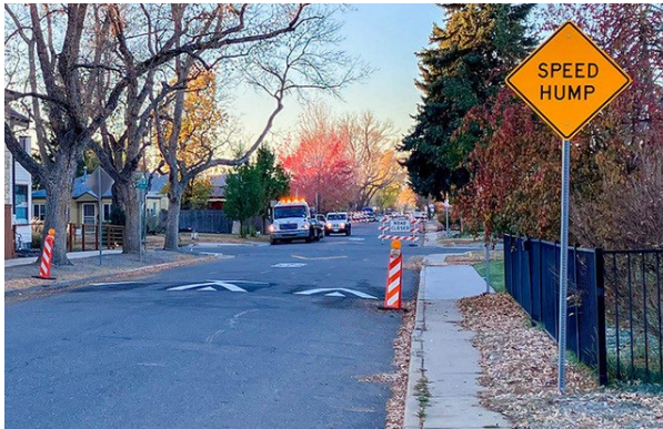
Speed cushion on North Perry Street in Denver (Source: DOTI)
